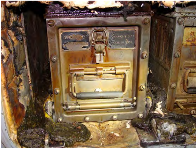
Fig. 13. The damaged 20NKBN-25 battery No 1 in the battery compartment of the Tu-154M RA-85684, which landed at Izhma airfield September 7, 2010 [8].
